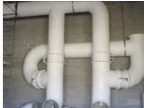
Prefabricated corrosion resistant duct system for water plant chlorine room
