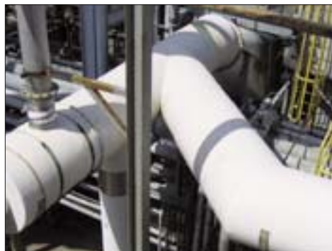
Prefabricated corrosion resistant duct system for water plant chlorine room
