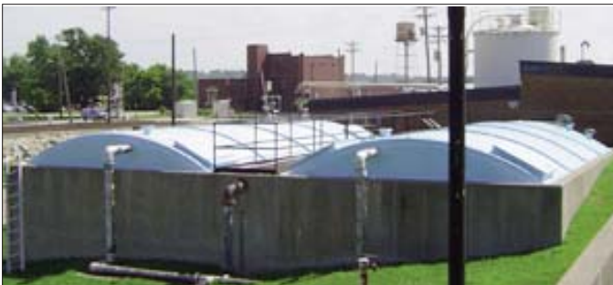
Tank covers, designed for snow and live loads
